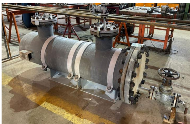
Heat exchanger after repair / maintenance
