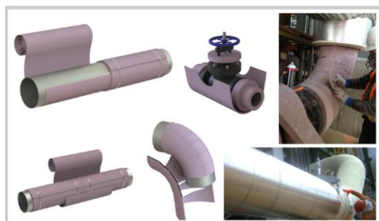
Figure 8. Installation of Pyrogel blankets on district heating pipelines
