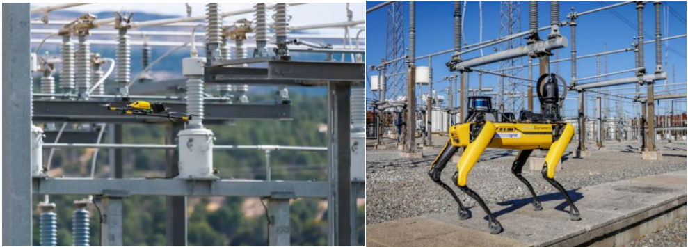
Figure 2. Inspection provided by robot / drone [4]
