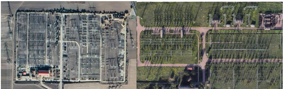
Figure 1. Aerial view of two different substations from Transelectrica’s grid
