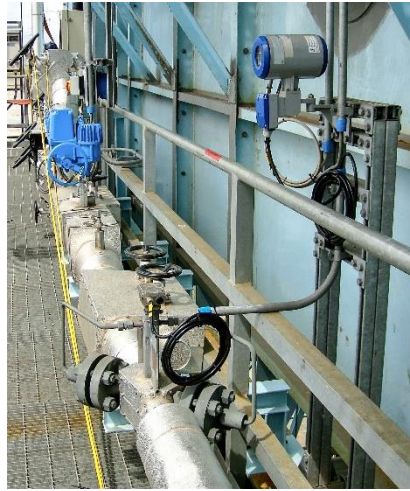
Figure 12. High pressure, high temperature Ultrasonic Steam temperature flowmeter for steam temperature water
