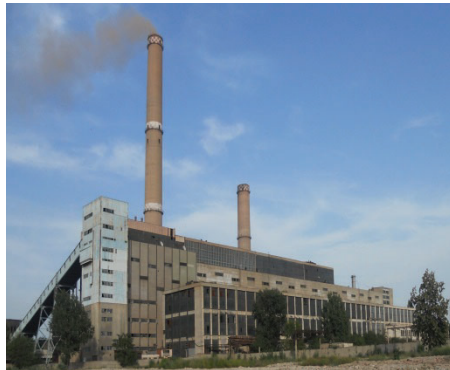
Fig. 1. Overview of the Western Cogeneration Power Plant of Oradea.
