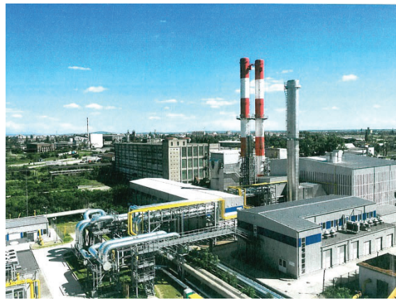
Fig. 19. Overview of the performant gas turbine installation manufactured by General Electric started up in 2016.
