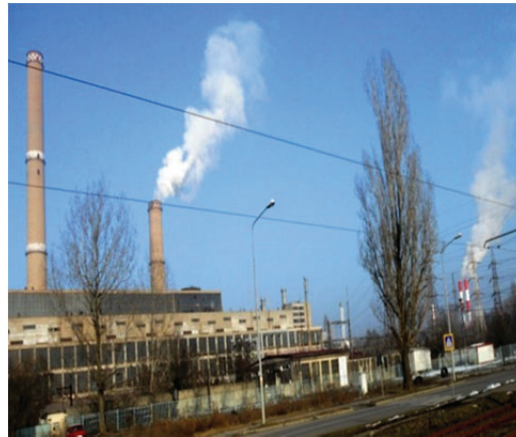
Fig. 21. Overview of the new thermal source operating in the western part of Oradea City from the winter 2016/2017 (new gas turbine installation together with the 25 MWe group upgraded on gaseous fuel).
