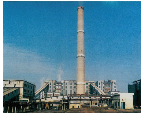
Fig. 2. Overview of the Eastern Cogeneration Power Plant of Oradea.
